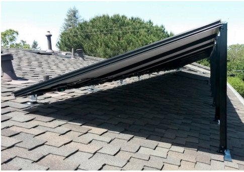
Figure 5-1 Reverse Tilt Picture and Schematic
