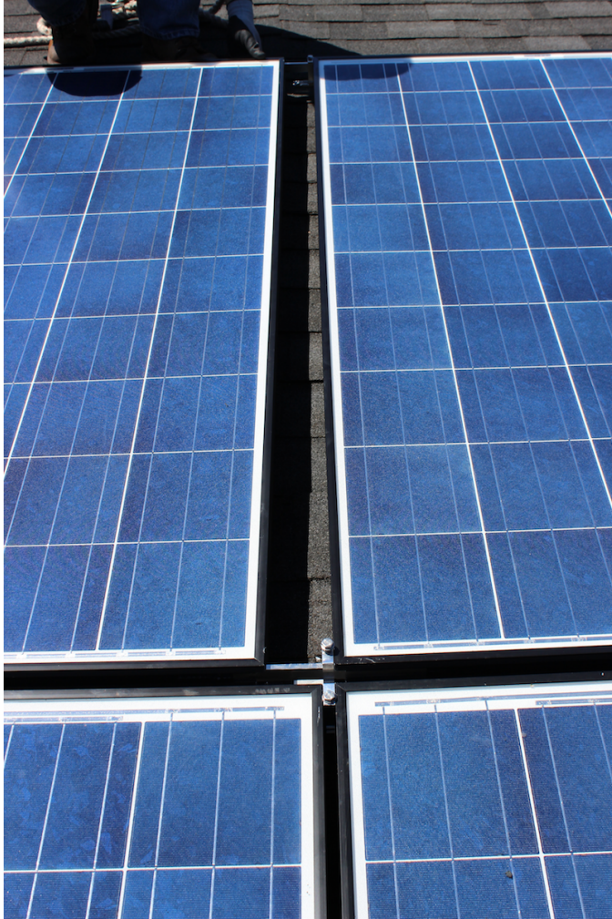
Figure 3-9 Installation of Third Module in Second Row
