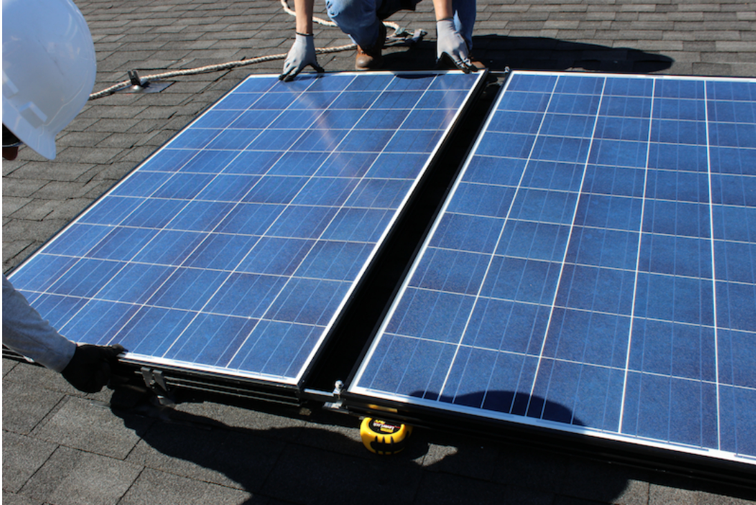
Figure 3-5 Installation of E-W Splices and Third Module
