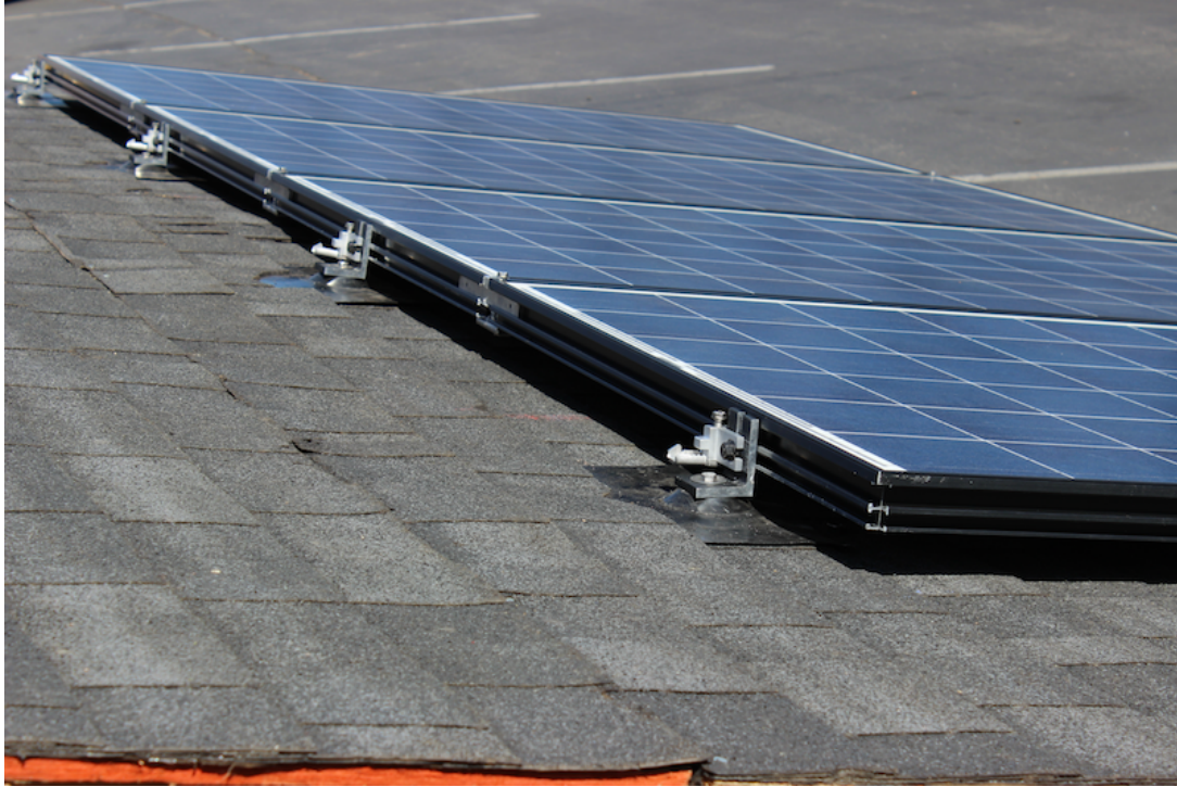
Figure 3-6 First Row of Modules Complete (With N-S Brackets)
