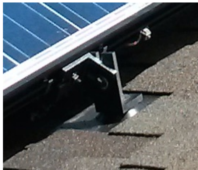
Figure 5-2 Reverse Tilt Ridge L-Foot Angle Adjustment, Bottom Back Leg, Top Back Leg
