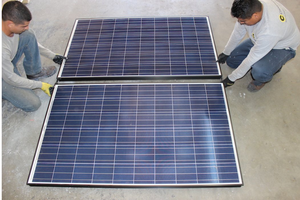
Figure 3-3 Pre-assemble First Two Modules
