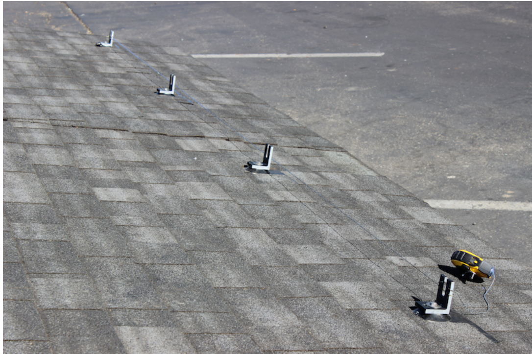
Figure 3-2 Align L-Feet on Bottom Row of Roof Mounts
