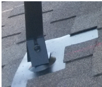
Figure 5-2 Reverse Tilt Ridge L-Foot Angle Adjustment, Bottom Back Leg, Top Back Leg
