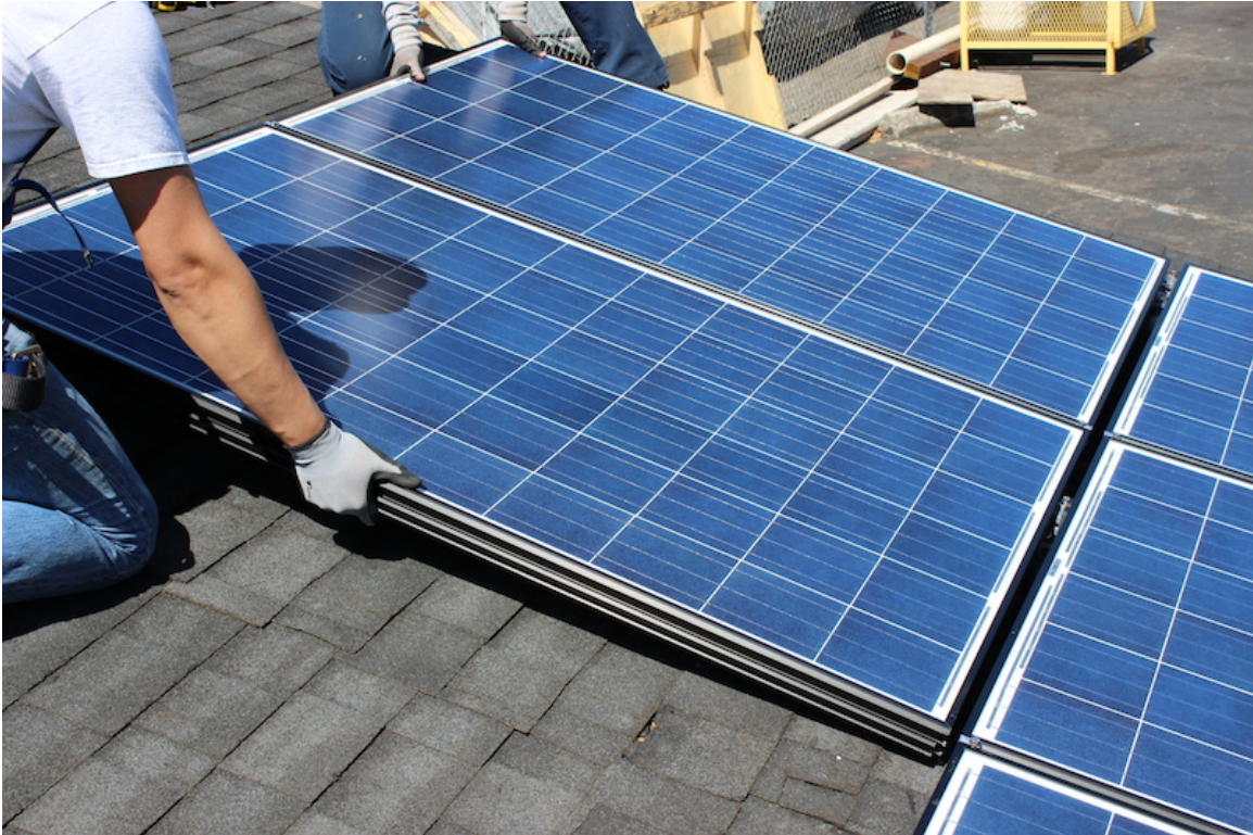
Figure 3-8 Installation of Second Row of Modules
